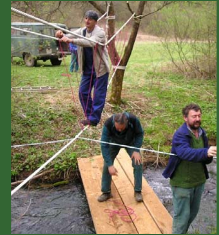
Image 72: Construction of the rope bridge in Aggtelek BR
